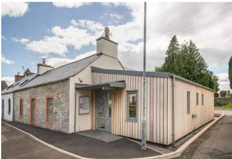
Balmaclellan Smiddy, Galloway: bringing a derelict building in the centre of the village back into use as a vibrant multi-use community centre , with electric vehicle charging (see section 4.7 below). More information in this video .
