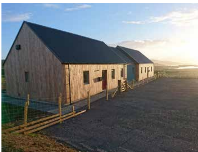
Ulva Ferry, Mull: affordable homes for locals , developed by the local community, where 10 years ago the local primary school was threatened with closure. More information in the SURF award citation from 2017 (see page 12 of the award brochure ).
