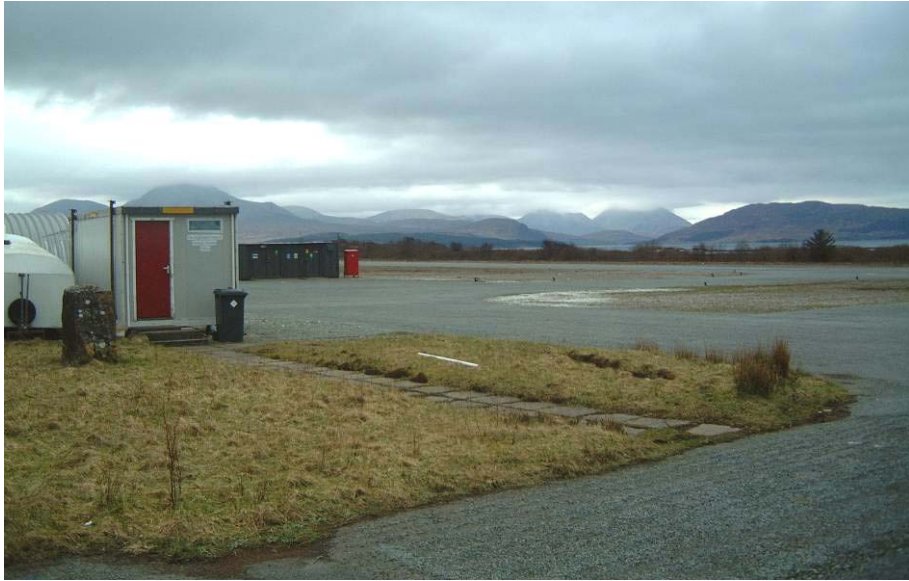
Figure 4 Existing Apron Area
