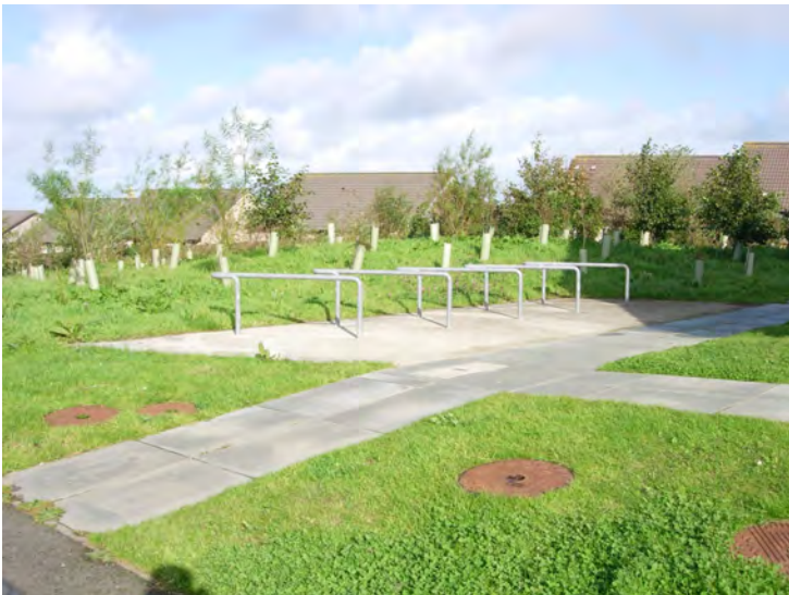
Residential cycle parking at new development at Ropewalk. Would benefit from a weatherproof cover.
