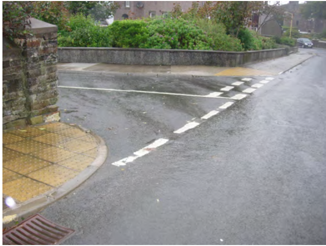
Good example of flush dropped kerbs and tactile paving on desire line at Buttquoy Crescent
