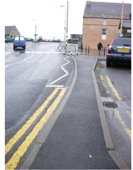
Narrow footway on Junction Road
