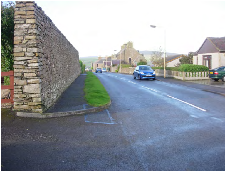
Grass verge should be removed on East Road to provide more space for pedestrians
