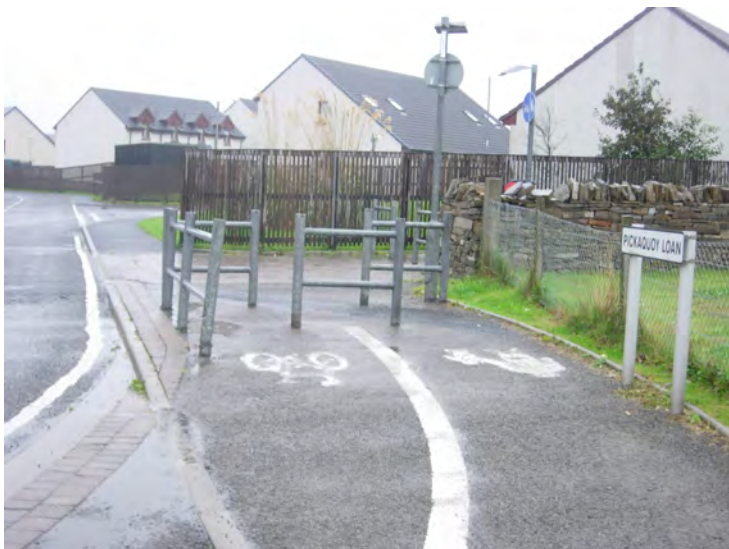
Over engineered access barriers
