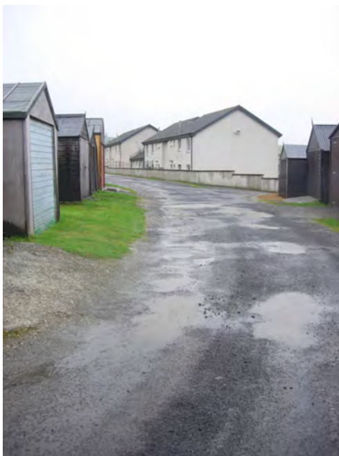
Shortcut through garages in Quoybanks should be surfaced and lit
