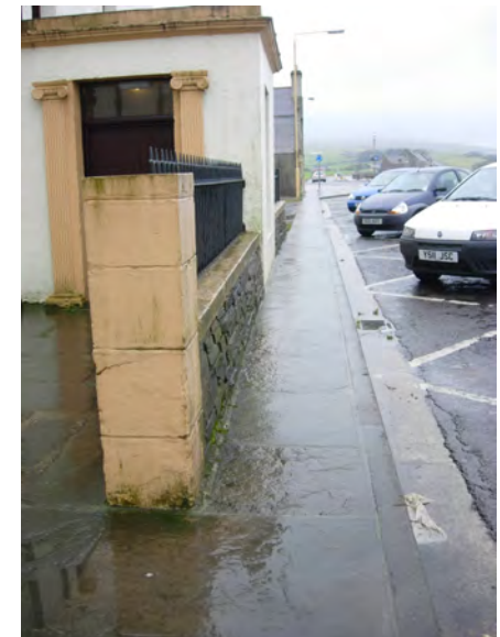
Narrow footway on Shore Street
