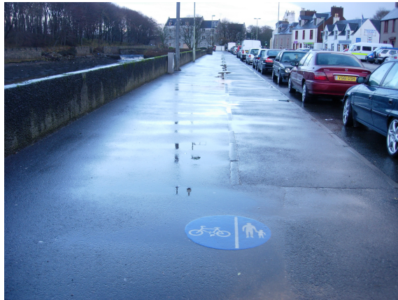
Figure 3-5: Segregated cycle track in Stornoway
