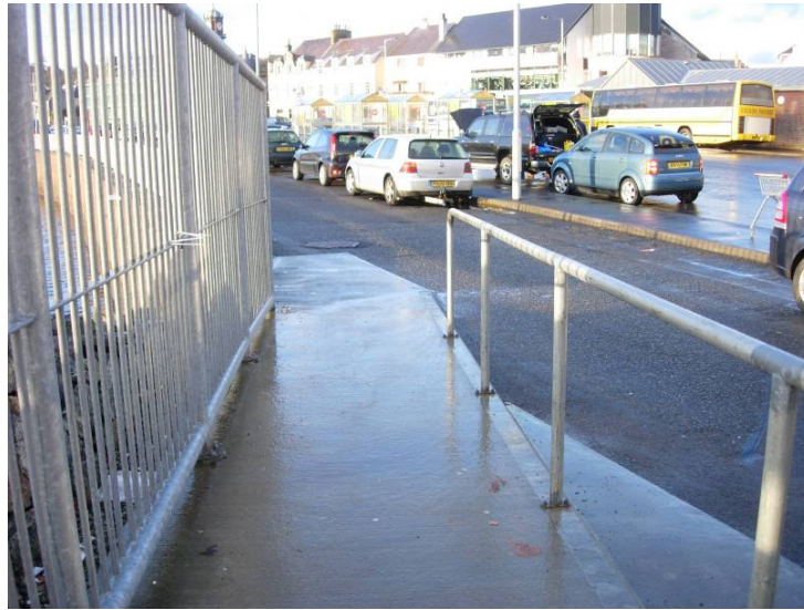
Figure 5-12: Pedestrian route from ferry has no continuity
