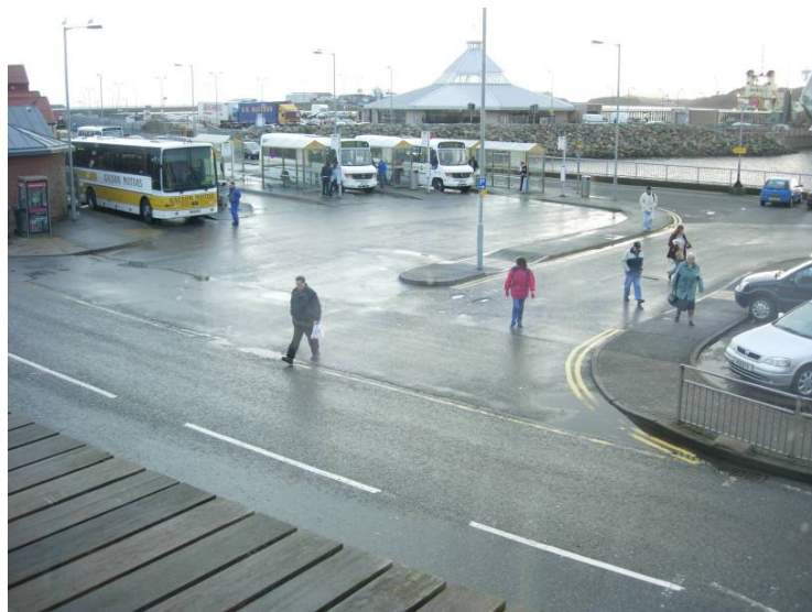
Figure 5-11: Lack of clear pedestrian routes
