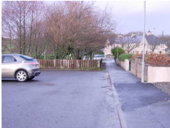
Figure 5-7: Road closure at Torquil Terrace/Macauley Road, could be improved by widening and providing dropped crossing
