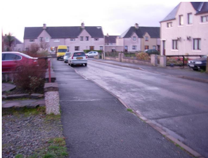
Figure 5-15: Typical residential road around Stornoway Primary
