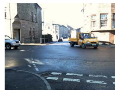
4A - Junction arrangement causes confusion for drivers and cyclists, options to improve layout should be investigated
