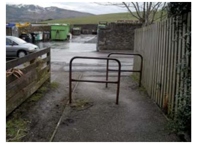
2A - Evident desire line at chicane feature for cyclists. Currently cyclists have to manoeuvre obstructive street furniture to use path and link onto Roding. Consideration could be given to providing a bicycle friendly feature which could involve resurfacing of approach path
