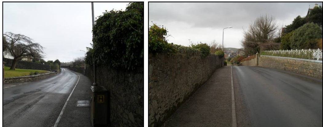
Figure 3.3: High walls and narrow footways along B842
