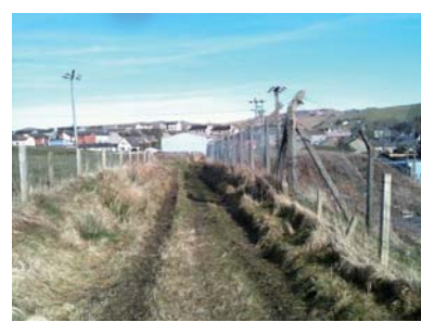
3B - Track would benefit from surfacing
