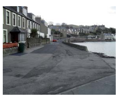
1E - Dropped kerbs and signage would assist navigation along North Shore Street with accompanying signage as is unclear if section is private access only
