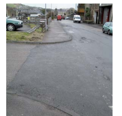
2C - The provision of dropped kerbs along Roding would improve permeability
