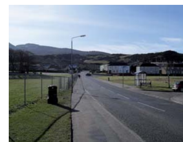
4D - Footway width is narrow along Ralston Road and Castlehill therefore an investigation of options to re-allocate road space to improve safety for pedestrians and cyclists, perhaps even an alteration to the road surfacing encouraging reduced vehicle speeds
