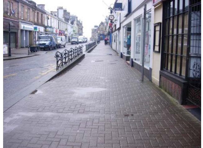
Figure 3.11: Wide footways in town centre
