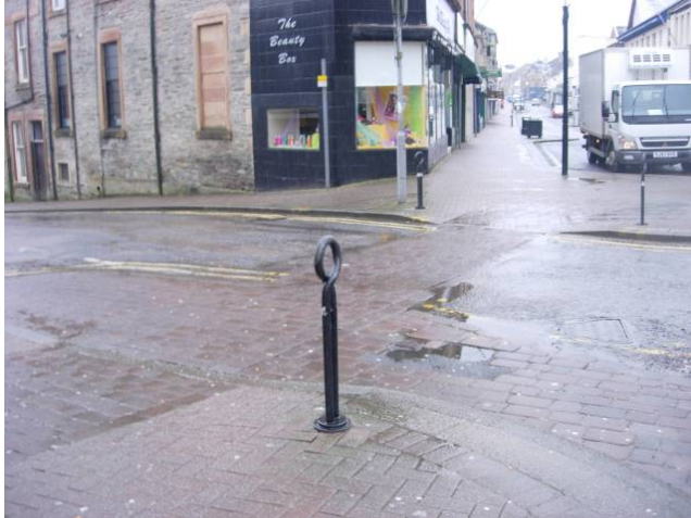
Figure 3.10: Flush dropped crossings in town centre
