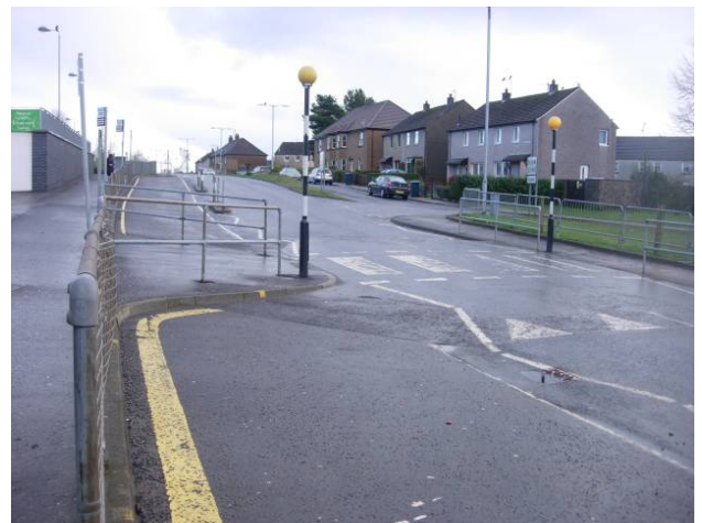
Figure 3.13: Raised zebra crossing at Dunoon High School
