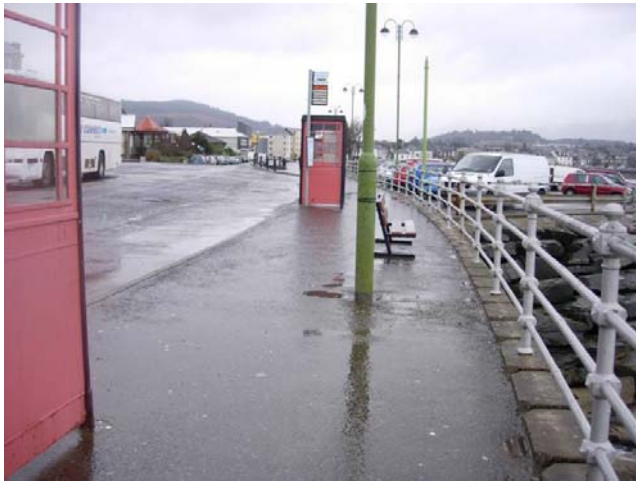
Figure 5.18: Promenade in town centre by bus terminal
