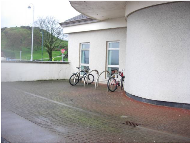
Figure 3.21: Cycle parking at ferry terminal
