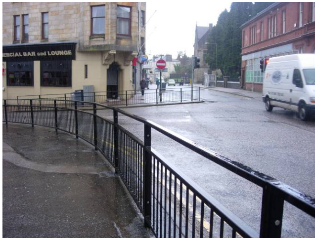
Figure 5.14: John Street, guardrail forces pedestrians away from desire line at signalised junction
