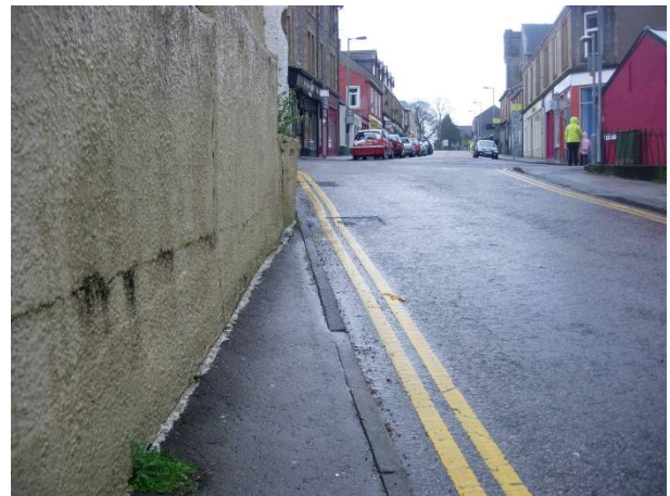
Figure 5.24: Narrow footway on Jane Street
