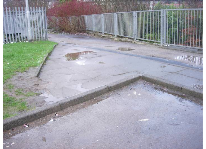
Figure 5.30: Need for dropped kerb at path to rear of St Muns Primary School
