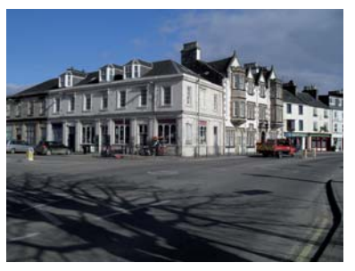
2A - No facilities for pedestrian crossing at the base of Argyll Street
