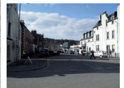
2C - Lack of dropped kerbs limits permeability for push chairs and wheelchairs
