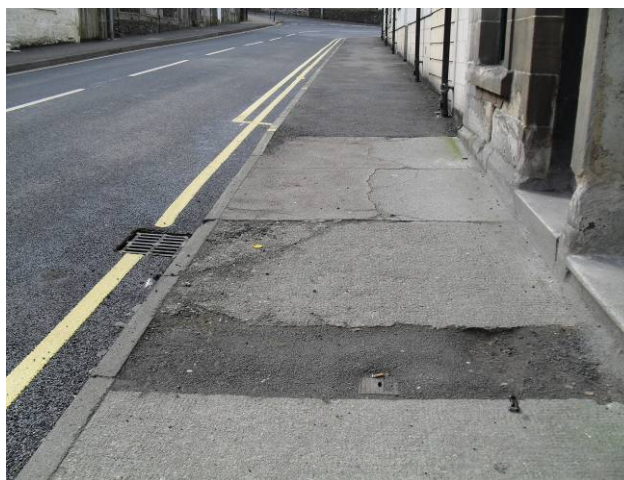
Figure 3.2: Inadequate surfacing on Bishop Street
