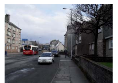
2G - Surfacing on both carriageway and footway is poor
