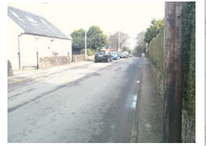
2E - Very limited width on footway causes a pinch point for pedestrians travelling to joint campus
