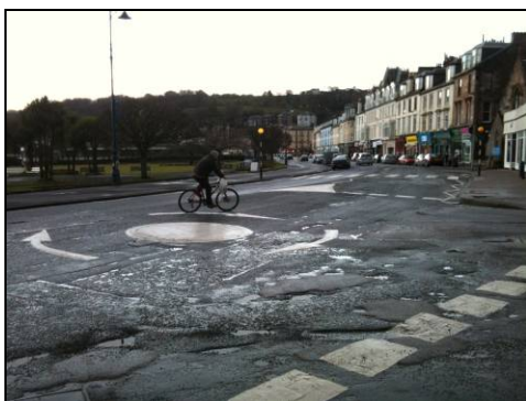
Figure 3.9: Damaged surfacing
