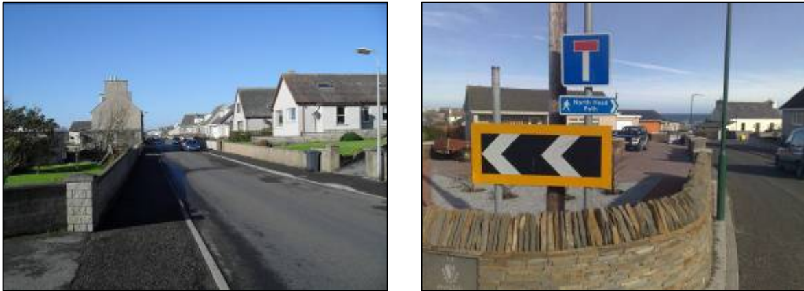
Figure 5-8: The link to Staxigoe is necessary to incorporate the settlement within Wick as it relies on the town for goods and services. The link also serves Hillhead Primary.
