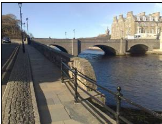
Figure 3-4: River Street with high quality paving and traditional street lights and Bridge of Wick in the background
