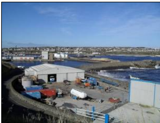
Figure 3-2: View from South Head Path looking back towards harbour
