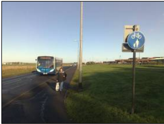
Figure 5-4: The northern section of the A99 currently provides a shared use path from Tesco toward Wick as far as Wick Industrial Estate. Wide roads and large junctions in northern section are not designed with active travel in mind
