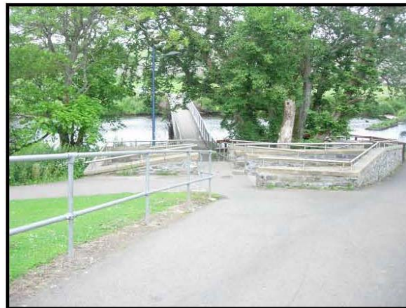
Figure 3.10: Access ramp on pedestrian bridge
