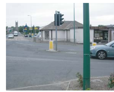
7g A number of pedestrian crossings are not signalled at the Bridgend / A9 junction.
