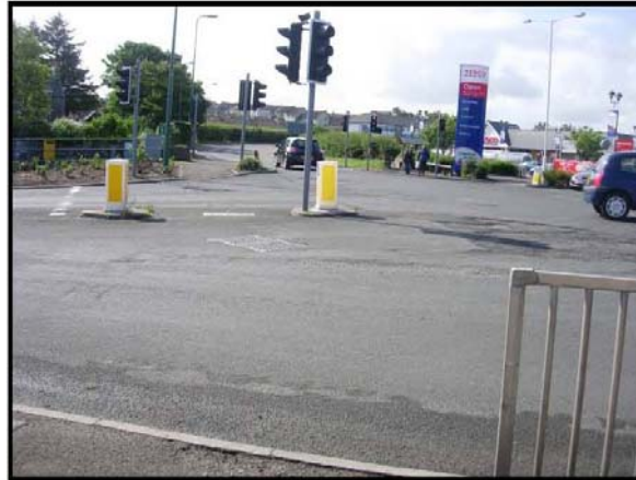
Figure 3.18: No pedestrian phase at signalised junction at supermarket
