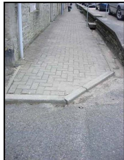
Figure 3.7: Typical footway detail in Thurso town centre: block paving with poor quality dropped crossings
