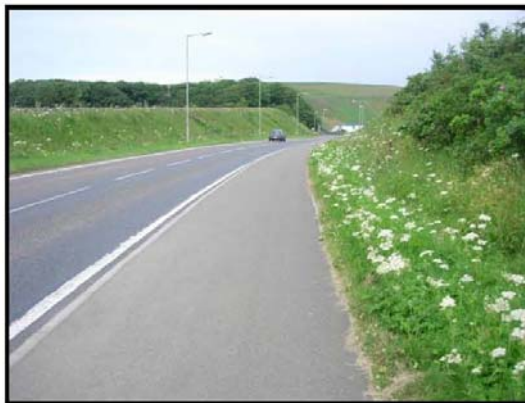
Figure 3.22: Wide footway on A9 to Scrabster Harbour
