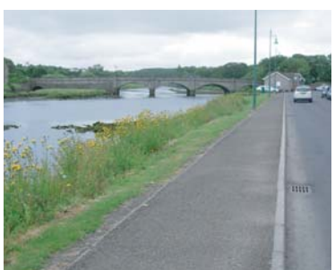
3f Riverside Road - part of 'circuit' for young drivers. Speed reducing measures may be needed pending further investigation.
