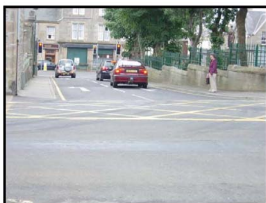
Figure 3.16: Gyratory system in town centre is not pedestrian friendly
