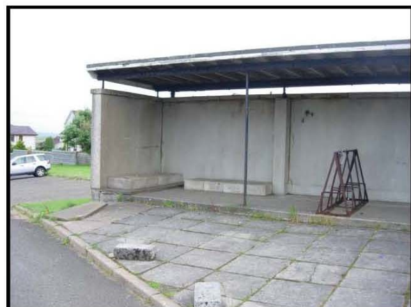
Figure 3.33: Poor quality cycle parking at North Highland College
