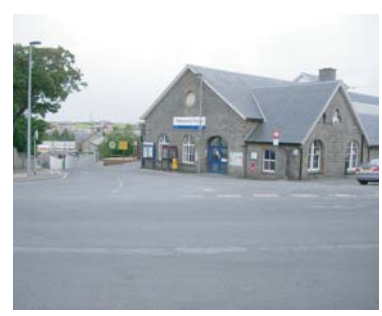
1b The junction at Castlegreen Road/Ormlie Road is very wide and intimidating for pedestrians.
