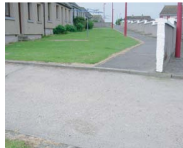
6d The existing track to Ormlie could be improved with the addition of dropped kerbs.
