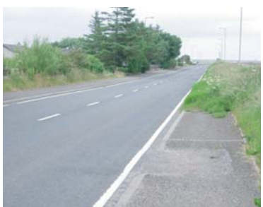
4c A shared use footway/cycle track is required on the A836 to the business park.
