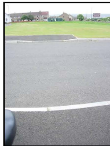
Figure 3.35: New dropped crossing with no tactile paving in new development
