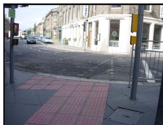
Figure 3.17: Pedestrian crossing to pedestrianised area
