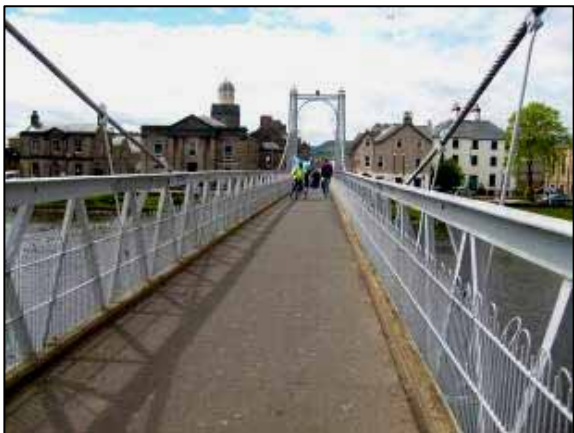
Figure 3-5: Pedestrian Bridge across River Ness
