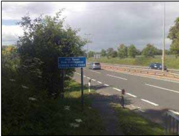
Figure 5-1: Current crossing of A9 at Beechwood connecting Inverness City Centre and out toward Culloden
