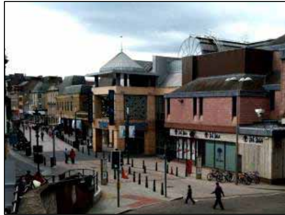
Figure 3-4: City Centre retail area
