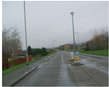
4h Existing informal crossing points could be made more conspicuous.
