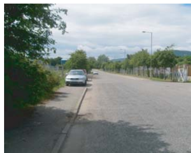
1i River Drive may require a segregated walking/cycling facility due to industrial traffic. Speed, volume and classification surveys are require.
