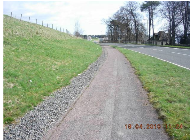
Figure 5-2: Existing footway between Alness and Belle Port
