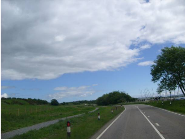
Figure 3-17: New footway on northern verge of B817
