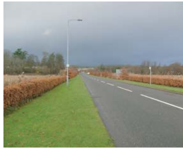
6a No footway on Teanich Avenue - a direct route to Alness Business Park.
