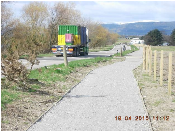
Figure 5-1: Newly constructed footway between Belle Port and Roskeen Bridge
