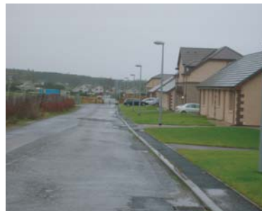
4k Inadequate footway in new build areas.
