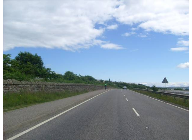
Figure 3-18: Cyclist making use of footway along B817 near Invergordon
