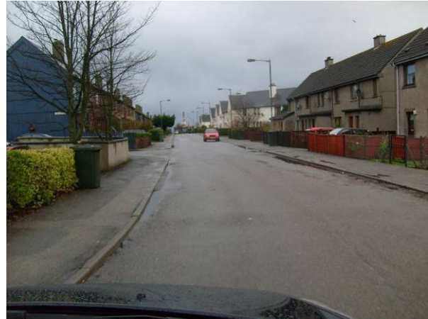
Figure 3-11: Typical residential street in Invergordon
