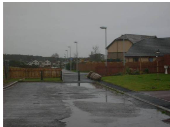
Figure 3-29: Pedestrian/Cycle link through road closure at Obsdale
