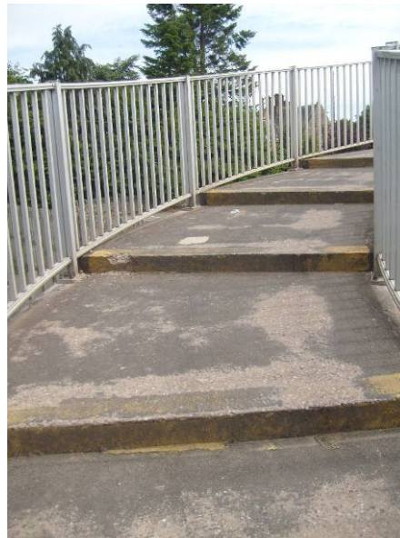
Figure 3-23: Stepped bridge over railway in Alness
