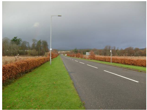
Figure 5-13: Bus stops on road linking A9 with Alness. Note lack of timetable/service information and basic pedestrian infrastructure such as pavements or crossings.
