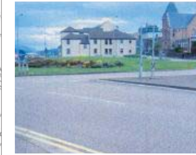
1m The roundabout at the end of the High Street is a difficult place to cross as a pedestrian. The roundabout is particularly forbidding for cyclists. More direct links are needed from Achintore Road to High Street.
