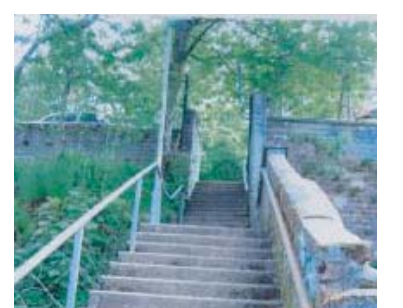
6a Handrail provision is good for each set of steps.
