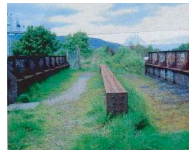
7b The bridge over the railway is still in place.
