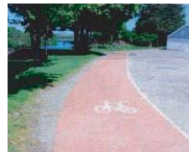
2c The designated route through the works club car park works well and is clear of parked cars.
