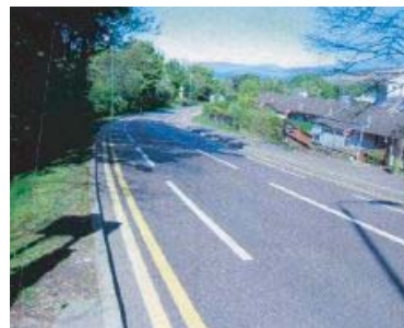
1d Other Local Authorities have been able to achieve reductions in speed by removing centre lines. See Appendix 2 for more information.
