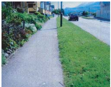
4a The northern side of the A830 from Corpach to Banavie lends itself to widening and conversion to footway/cycle track. The majority of housing is on the side of the road. A good quality crossing point will be needed to access the local shops, Banavie Primary School and the Fort William Spine Route via Station Road.
