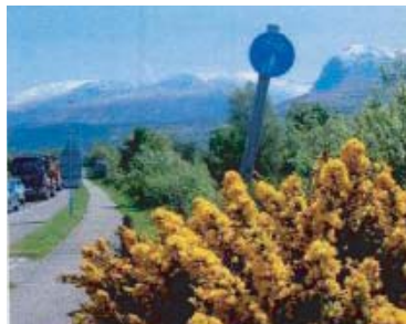
4c The existing cycle tracks on the A630 from Banavie Station to the junction of Lochaber High School would benefit from regular maintenance.
