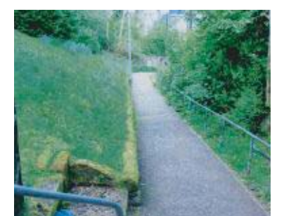
6b Parts of these well used steps to the town centre are not overlooked and may benefit from installation of CCTV.
