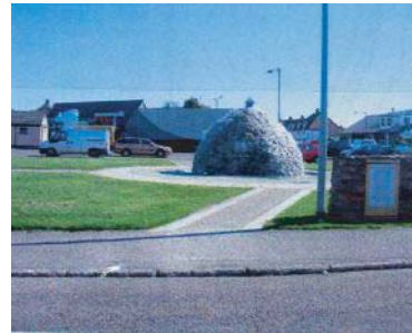
1b The installation of flush dropped kerbs would improve access to local shops from the spine route/Great Glen Way.
