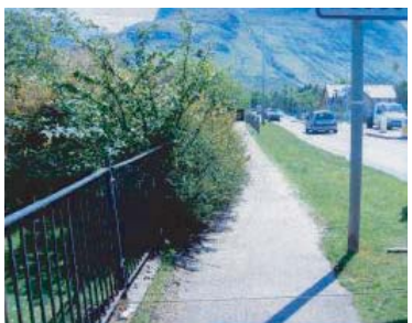
4c The existing shared use facilities on the A830 should be extended to the A82 with improved crossing facilities at the junction to the high school and health centre. The tracks should connect with the cycle route to Toriundy.
