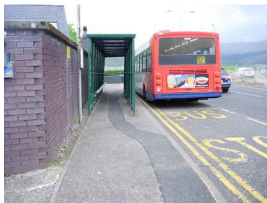
Figure 3-24: Inadequate bus stop provision for services into Fort William
