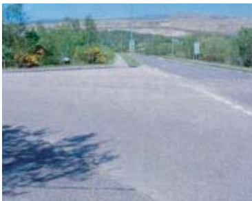
4b The junction for Blar Mhor Industrial Estate on the A830 is very wide and leaves pedestrians and cyclists very exposed. One solution could be the introduction of "Elephants footprints" to highlight the presence of the cycle route.
