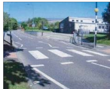
1d Bus drivers tend not to use layby to allow passengers to alight. Area could be redesigned to provide safer bus stop provision.
