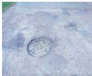
2a The carriageway adjacent to the house at Inverloch Castle can be particularly hazardous for cyclists, especially in the dark.
