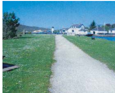
1a Route from Corpach Locks to existing track has stone to dust surfacing and is relatively good quality, but gravel forecourt from Station Road to Locks is difficult to cycle on.
