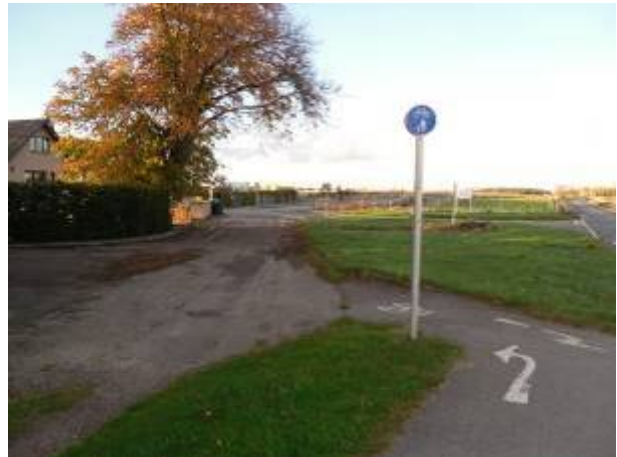
Figure 5-62: Poor design of transition with faded surface markings
