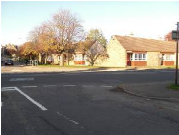
Figure 5-26: Wide junction radius typical of side streets on Orchard Road
