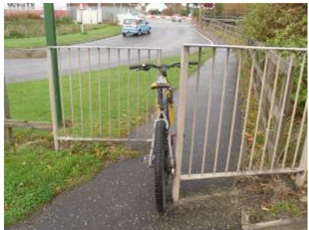
Figure 5-11: FSN 2 Narrow chicane restricts cycle access to NCN
