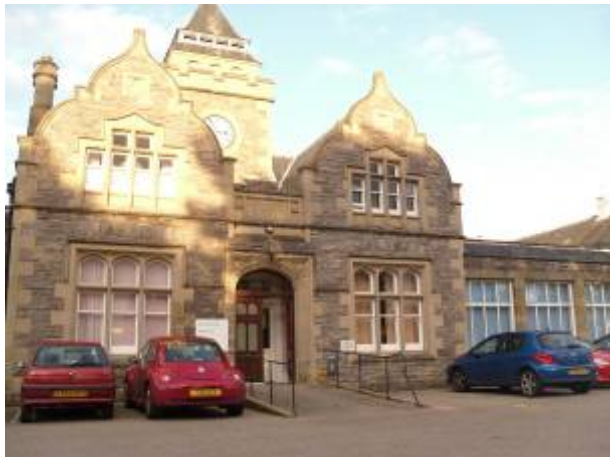
Figure 5-38: FSN 6 Leancoil Hospital on the south east side of Forres
