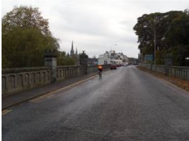
Figure 5-8: FSN1 Cycle lanes on Bridge Street come to abrupt end when entering the retail centre
