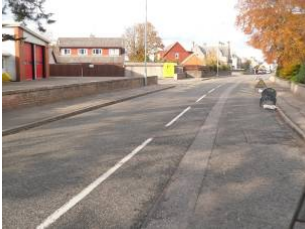
Figure 5-30: FSN 4 Road tightens near junction with Fleurs Place
