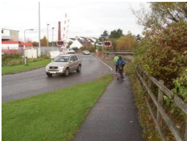
Figure 5-10: FSN 2 No provision for cyclists at level crossing
