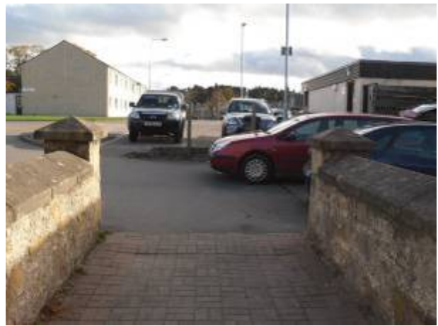
Figure 5-47: Good pedestrian link blocked by parked cars and step
