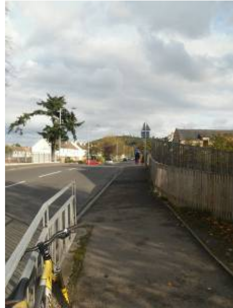
Figure 5-25: FSN 3 Footway narrows as Orchard Road heads east
