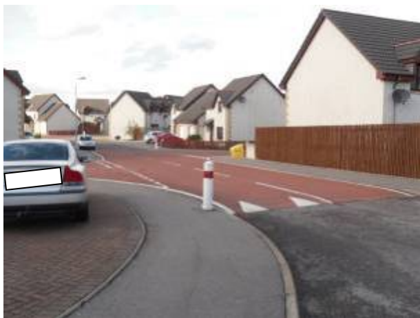
Figure 5-56: Example of existing traffic calming in new residential area at Knockomie
