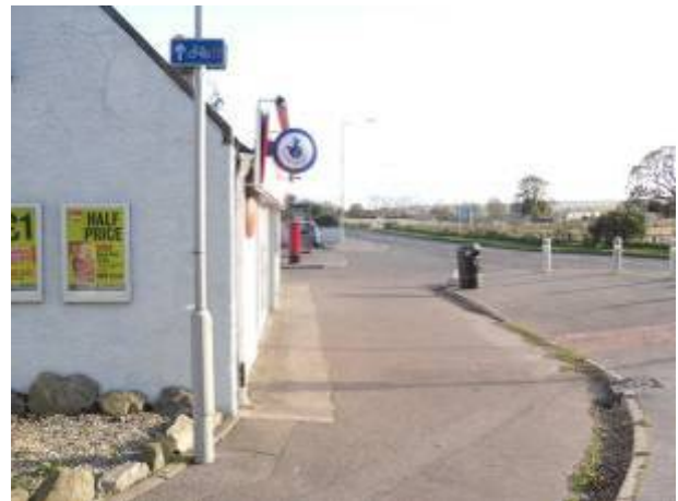
Figure 5-41: Kinloss shops with wide footway although limited safe access from main housing areas on south side of road
