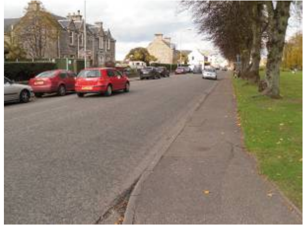
Figure 5-31: FSN 4 Wide area from Orchard Road to Bridge Street Roundabout
