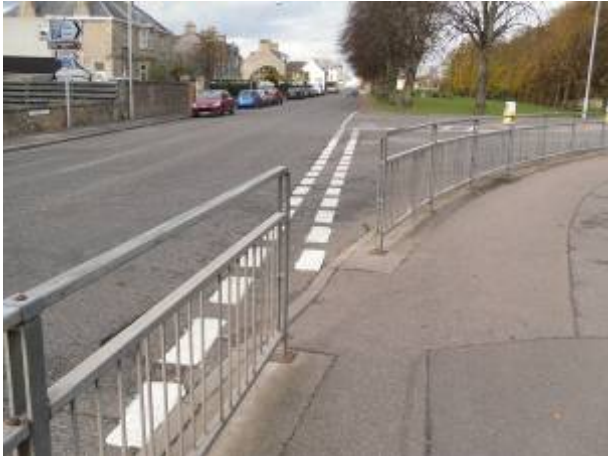
Figure 5-24: FSN 3 Access point to Orchard Road restricted by guardrail
