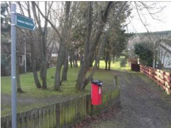
Figure 5-21: Aviemore Orbital Path requires upgrading
