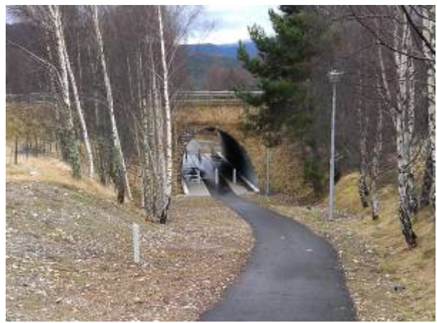
Figure 3-24: High quality traffic free link under A9 from High Burnside
