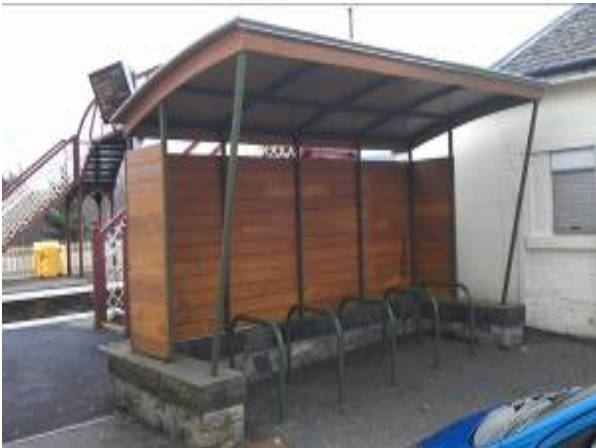
Figure 3-25: Cycle parking at Aviemore Rail Station
