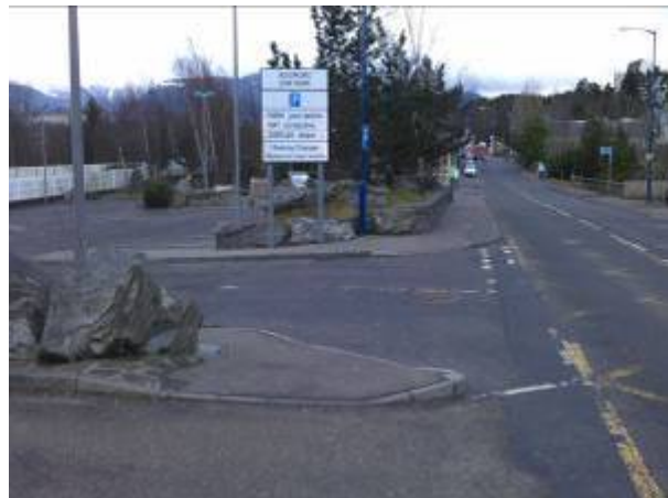
Figure 5-2: No tactile paving, dropped kerbs to be flush
