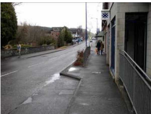
Figure 3-11: Footways at some locations are narrowed by the provision of on street car parking
