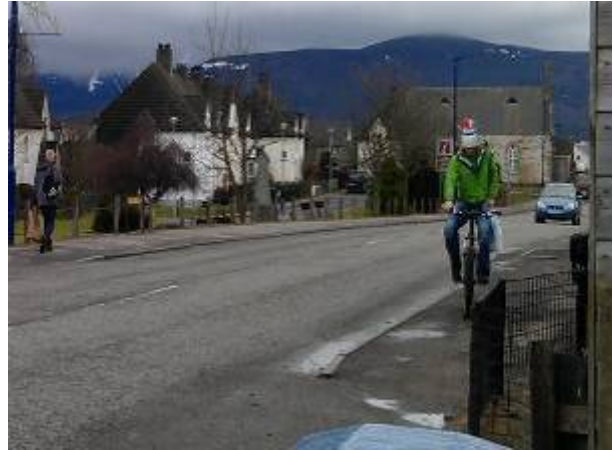
Figure 3-22: Narrow footways on some areas of Grampian Road are still used by some cyclists
