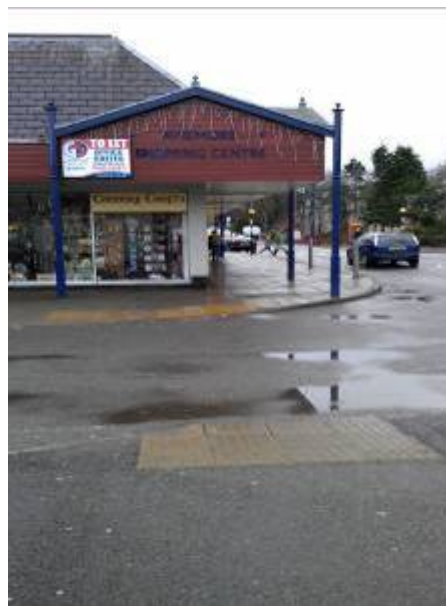
Figure 3-10: Example of tactile paving in Aviemore town centre, generally not provided throughout settlement
