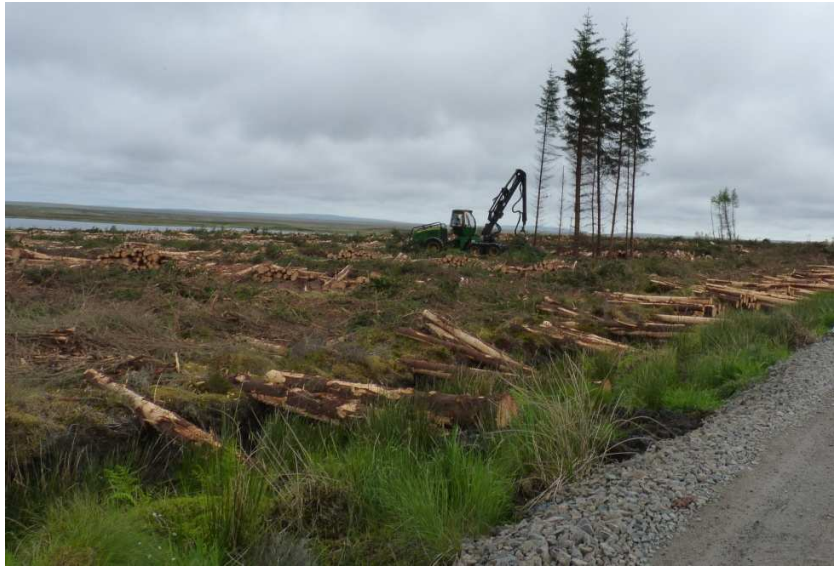
Picture 1: Picture 2 Flow Country peatland restoration proceeding using Braehour Link
