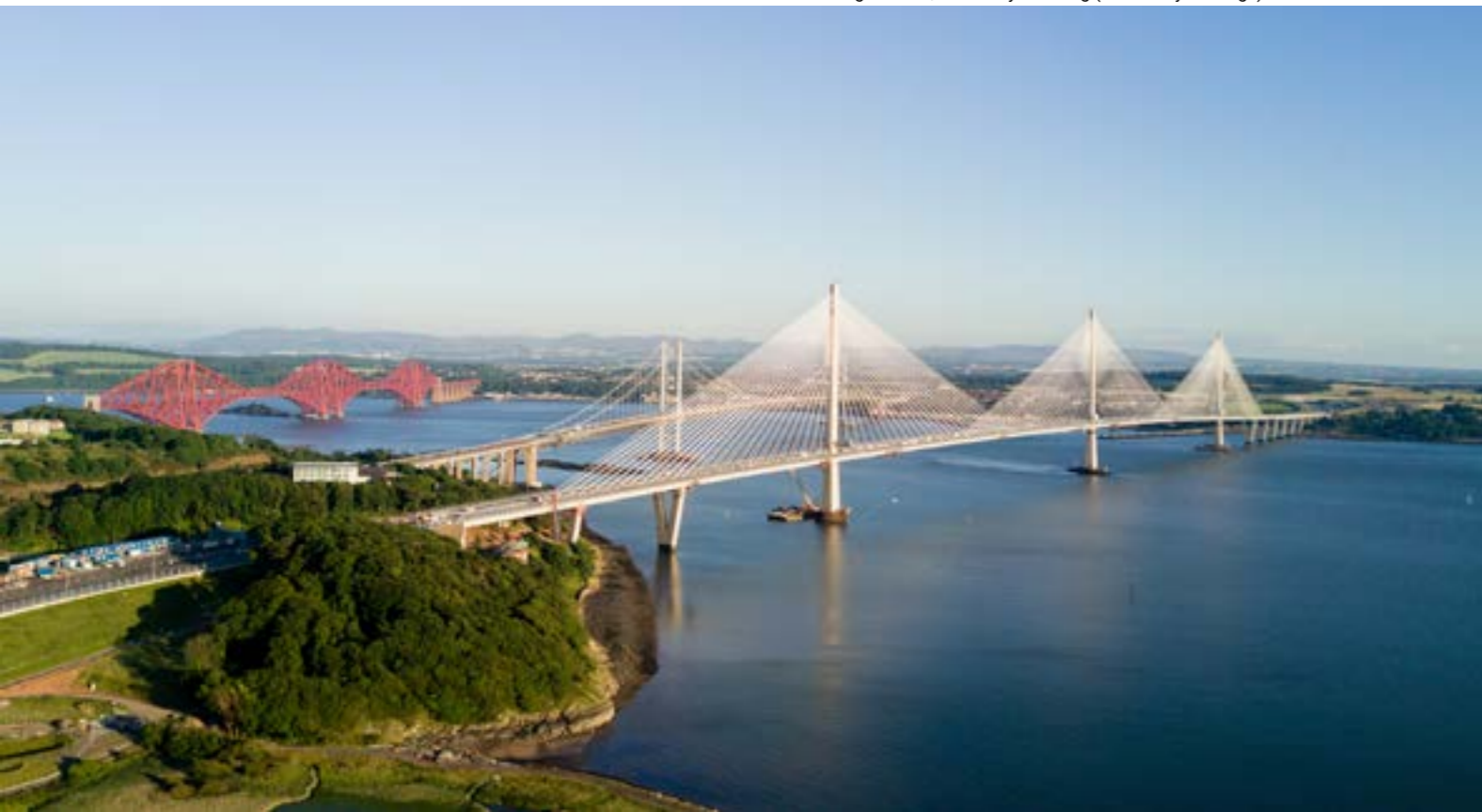
Figure 17: Queensferry Crossing (Cable Stayed Bridge)
