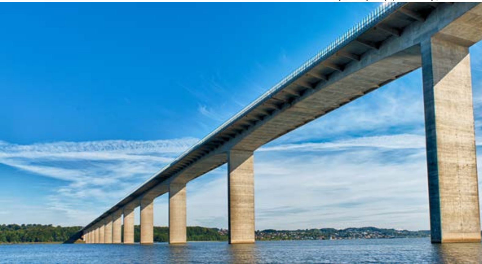
Figure 21: Vejle Bridge (Cantilever Bridge)
