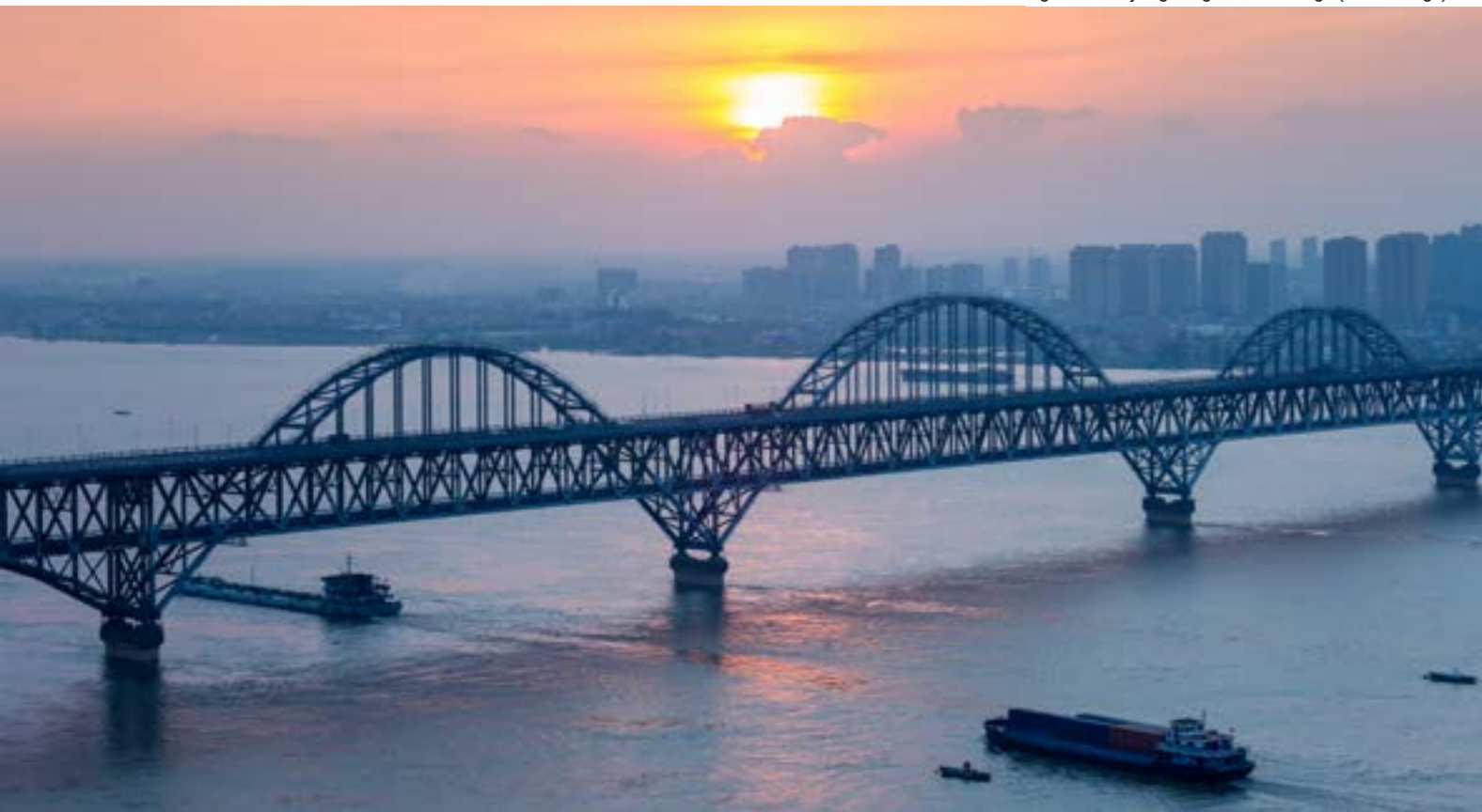
Figure 22: Jiujiang Yangtze River Bridge (Truss Bridge)
