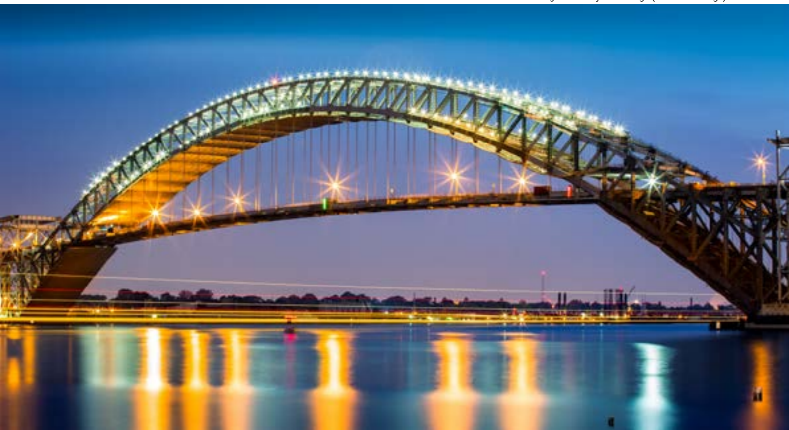
Figure 19: Bayonne Bridge (Tied Arch Bridge)
