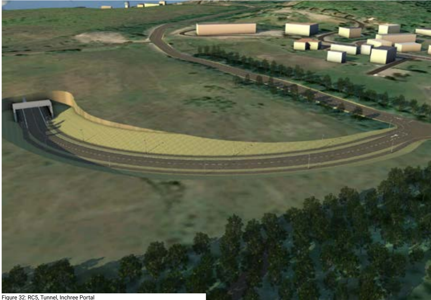
Figure 32: RC5, Tunnel, Inchree Portal
