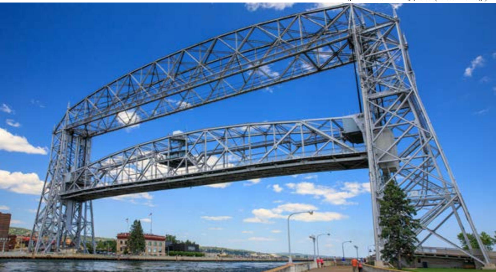
Figure 20: Aerial Lift Bridge, Duluth (Vertical Lift Bridge)
