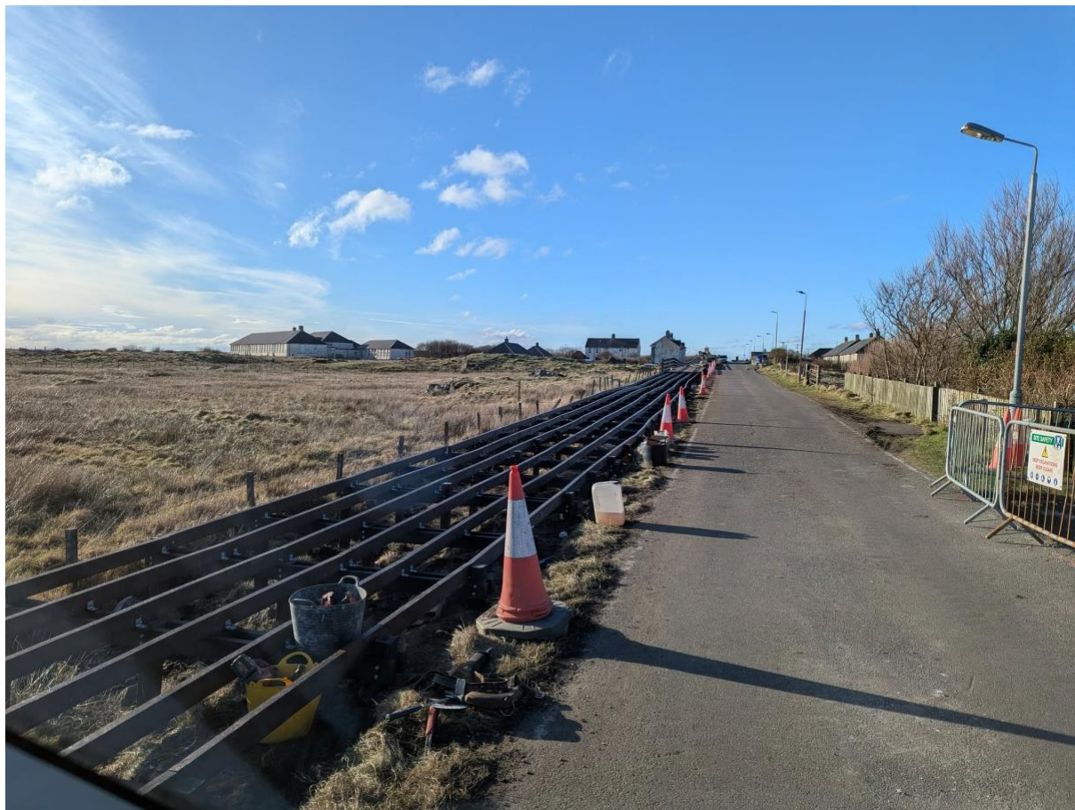
Path under construction – January 2026 – looking towards school (top left)
