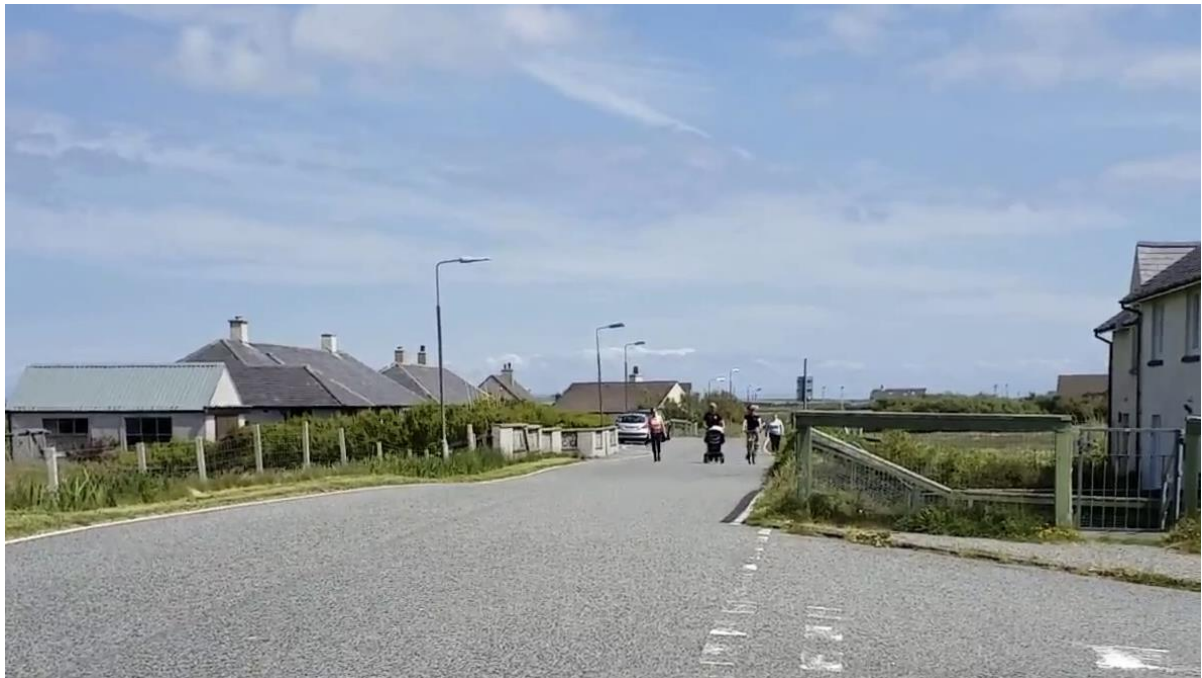
There was no footway through lochdar, on a national speed limit road
